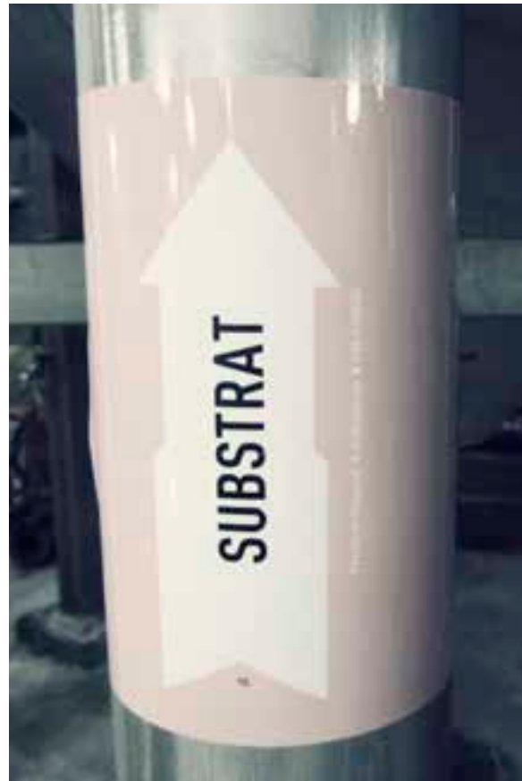
There are many advantages with a clean substrate: increased gas exchange, optimized use of space in digesters, and less wear on the machinery.
