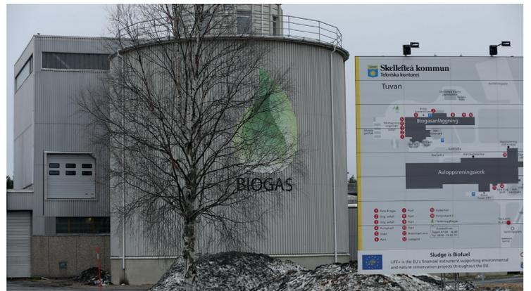
Contrary to the Swedish "co-digestion" terminology used, Tuvan's food waste biogas plant is a co-located facility and separate from the WWTP. Shared facilities, biogas storage, upgrading, compression and flare are all post-digestion.
